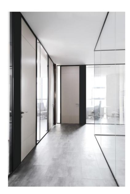
Panorama means without any visible frame between glass and glass on the sizable glass wall, which is able to maximize visibility within limited space.
